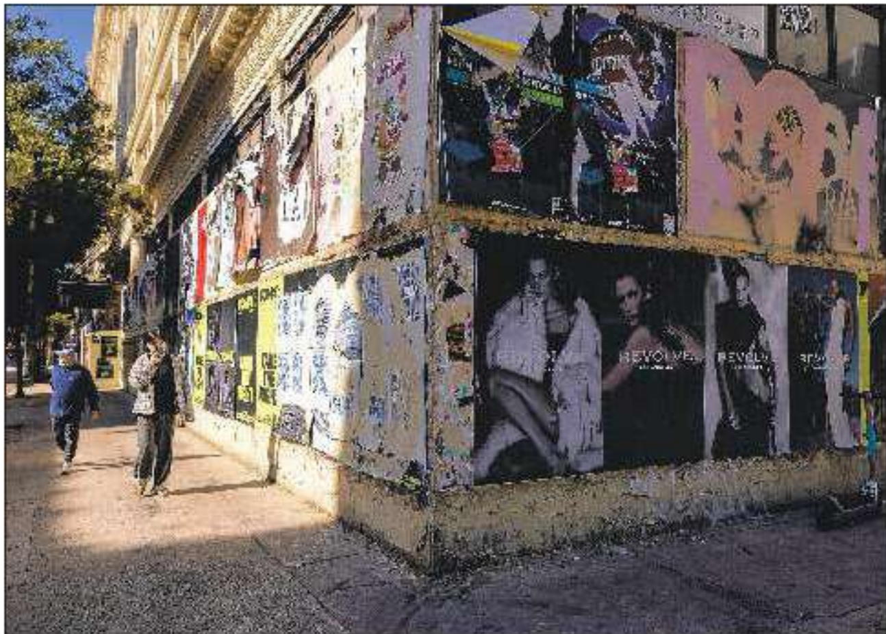
FIRMS have left downtown for more vibrant L.A. areas. Above, a boarded-up building on Broadway.
