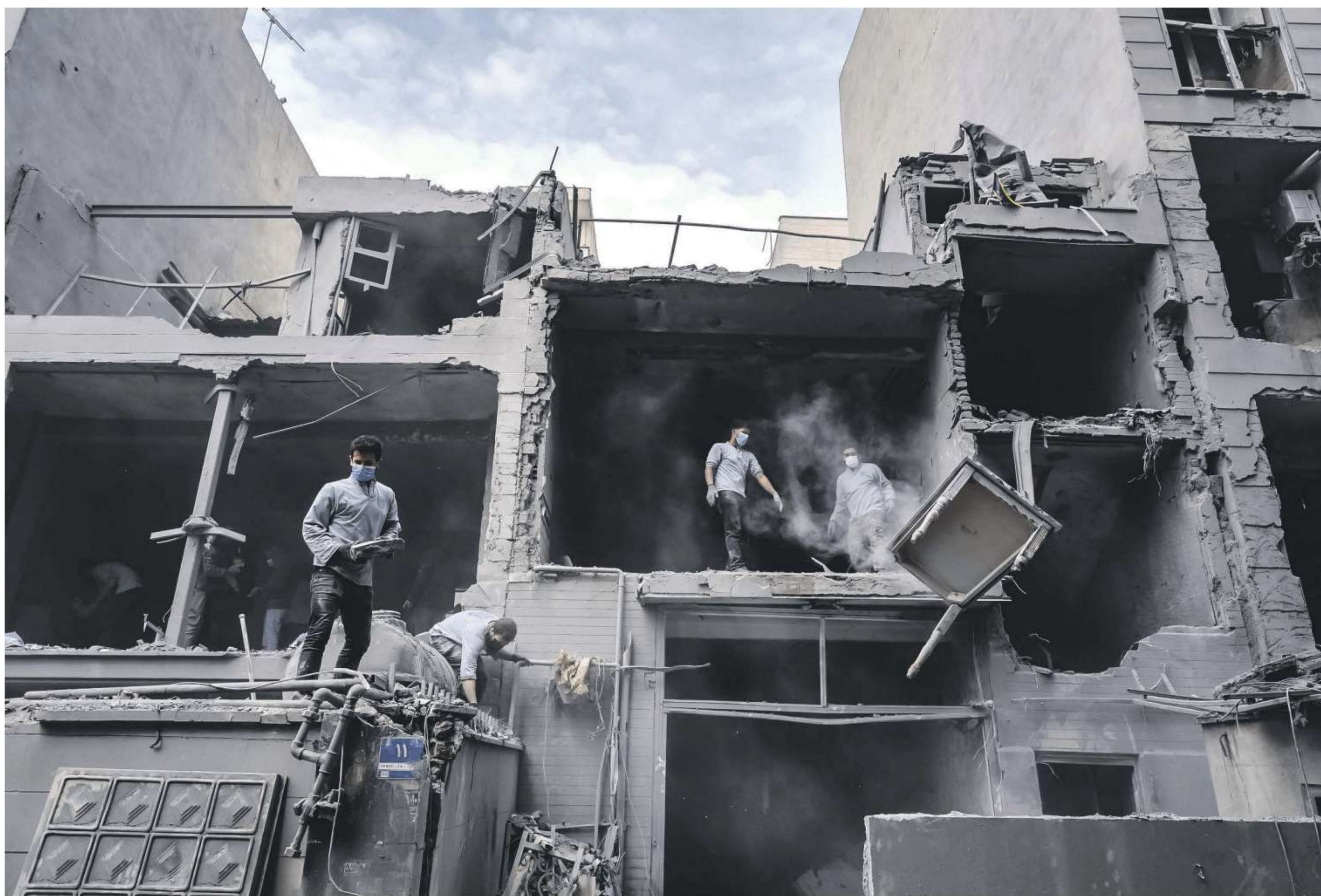
▲ Volunteers work in Tehran yesterday to clear debris from a residential building damaged in a strike on a nearby police station PHOTOGRAPH: VAHID SALEMI/AP
